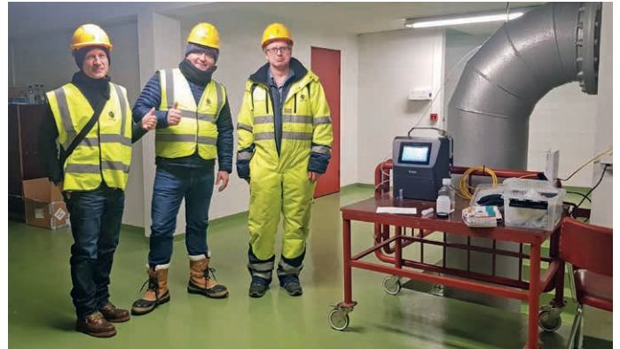
Figure 2: Installation of BactoSense
