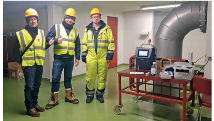
Figure 2: Installation of BactoSense
